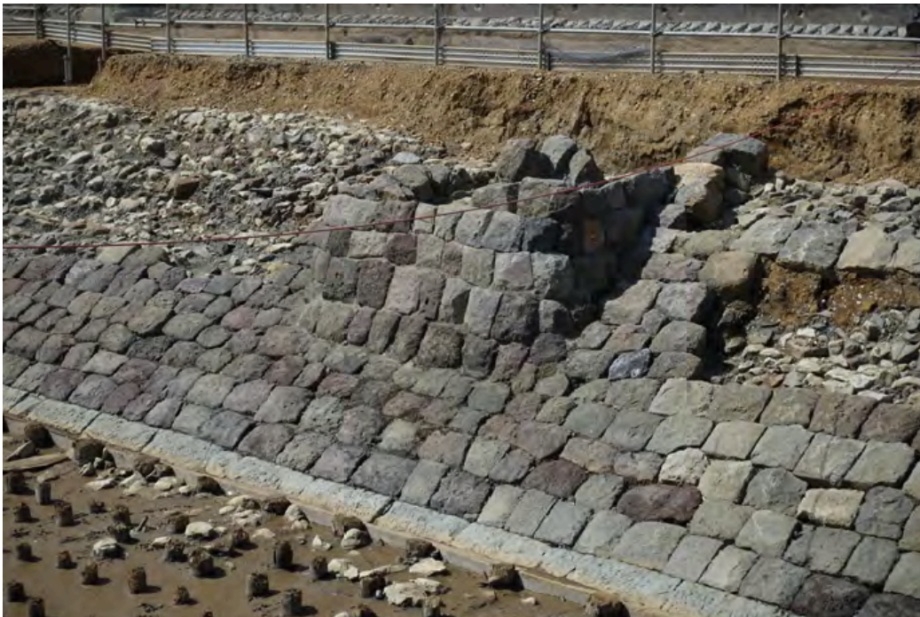
The protrusion of what appears to be a signal box
